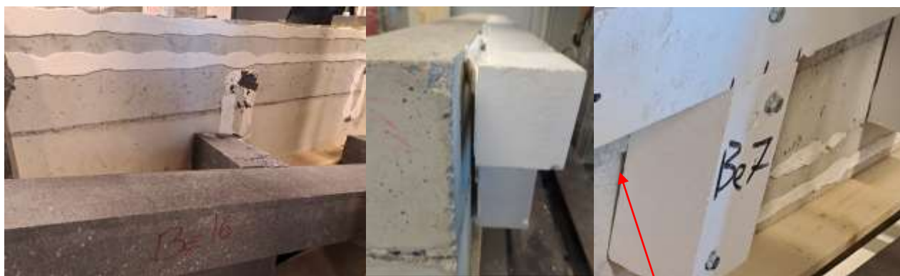
Fig. 13. CONCRETE wall construction after tests. Tolerance flaws.
