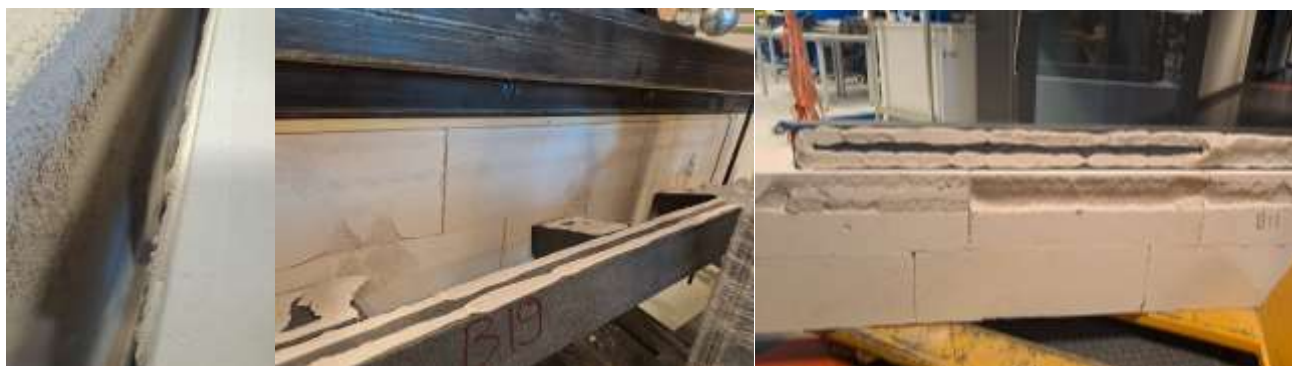
Fig. 7. BAUROC wall construction after tests.
